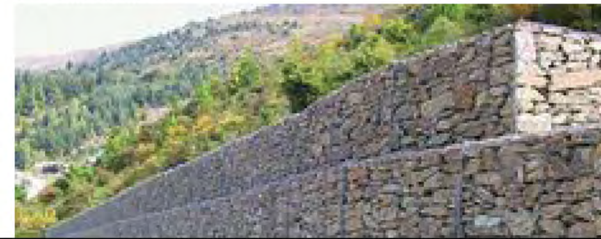
⑩ Gabion Walls
