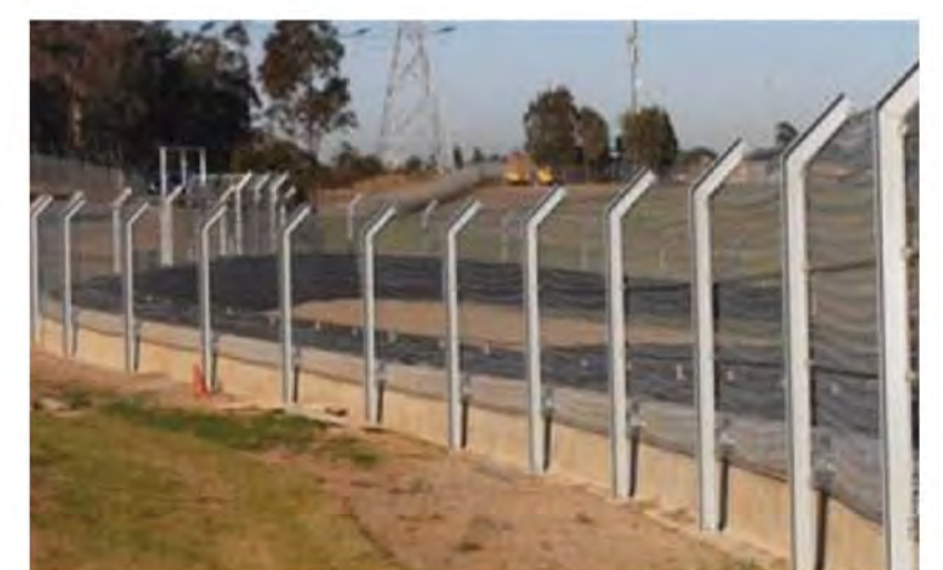
Catch Fence on the top of Barrier Fence
